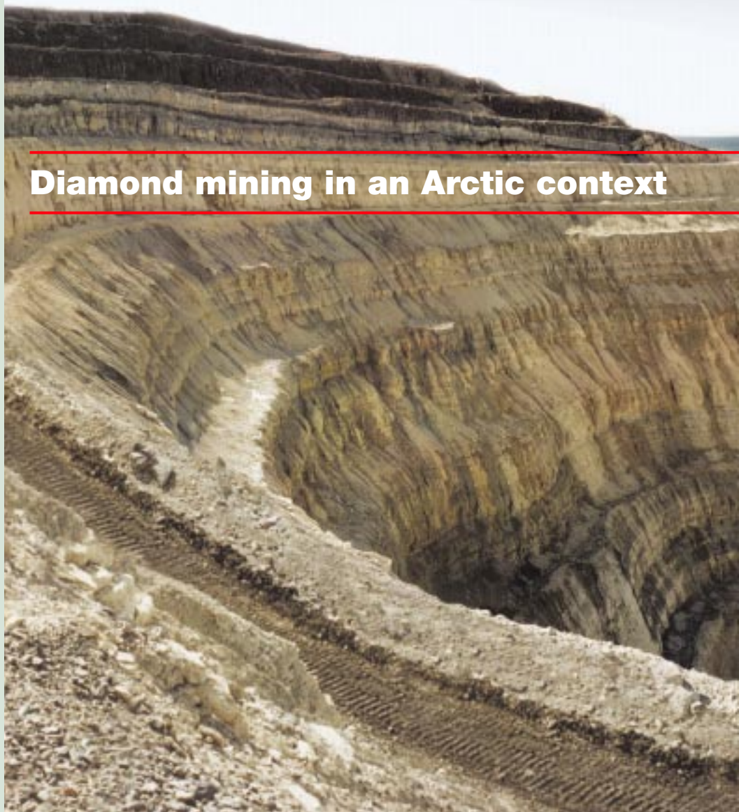
Steep slopes of Aikhal diamond mine are only feasible because of permafrost.
